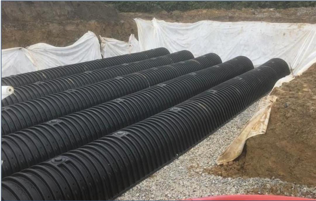
Plate 3-3 Typical Poly-Tunnel Installation Arrangement
